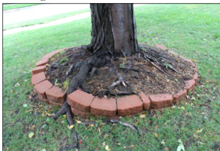
Shallowed rooted tree breaking through block edging.
