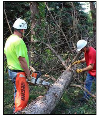
Jeff & Jason working hand in hand during a tree removal.
