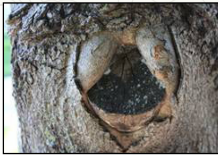
Improper pruning cut into the branch collar.
