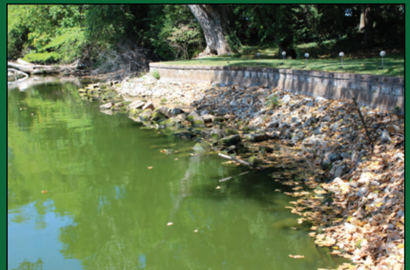
The water table has been lowered way below the top of the wall because of the 2020 drought.
